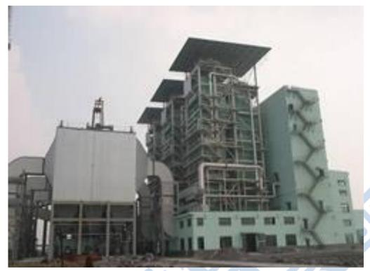
Circulating fluidized bed power station boiler
