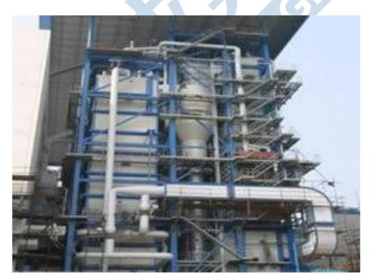
• QXX high speed external circulating fluidized bed boiler
