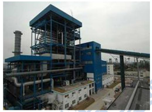
QXX low speed internal circulating fluidized bed boiler
